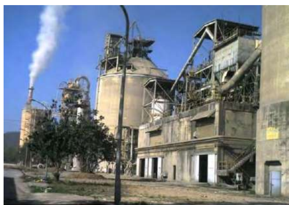
Fig: Udaypur Cement Industry
